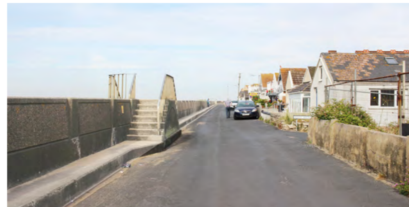
Fig. 75. Photograph of current condition of Brooklands
