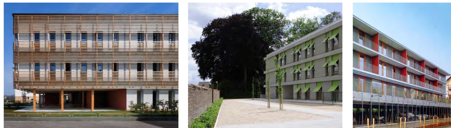
Fig. F6. Examples of good quality, well-designed 3-storey homes with non-habitable ground floor
